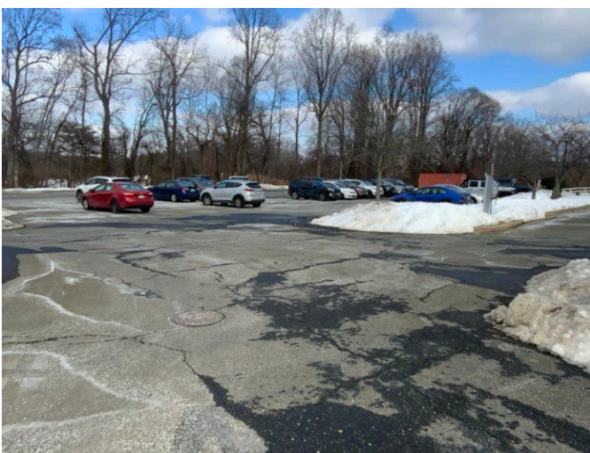
23 - PARKING AREA OVERVIEW
