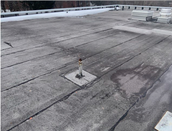
7 - MODIFIED BITUMINOUS ROOFING
