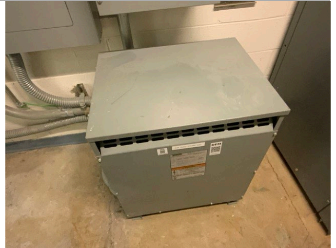
20 - SECONDARY TRANSFORMER
