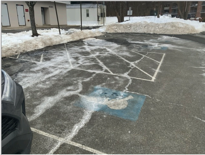
OVERVIEW OF ACCESSIBLE PARKING AREA
